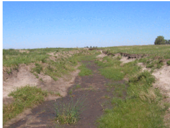
Site where water control structure will be placed in existing drainage ditch.
