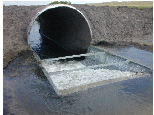
Weir installed on existing 10-ft diameter tube.
