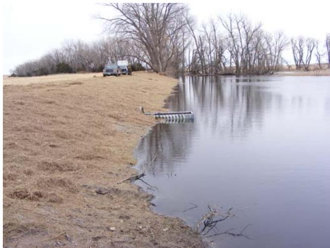
What is not visible in this photo is a second water control structure located where the vehicles are parked. The foreground structure serves as an emergency overflow structure. The second structure controls normal flows and allows the owners to divert some of the runoff onto a large meadow.
