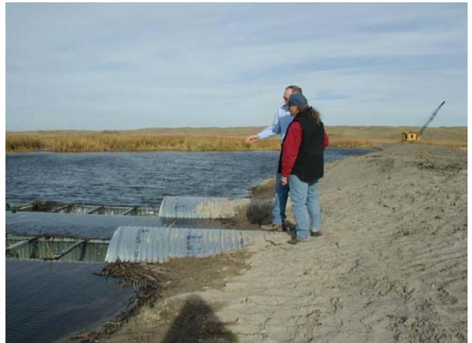
**Figure 1 Twin-tube water control structure on Wolfenden.**
